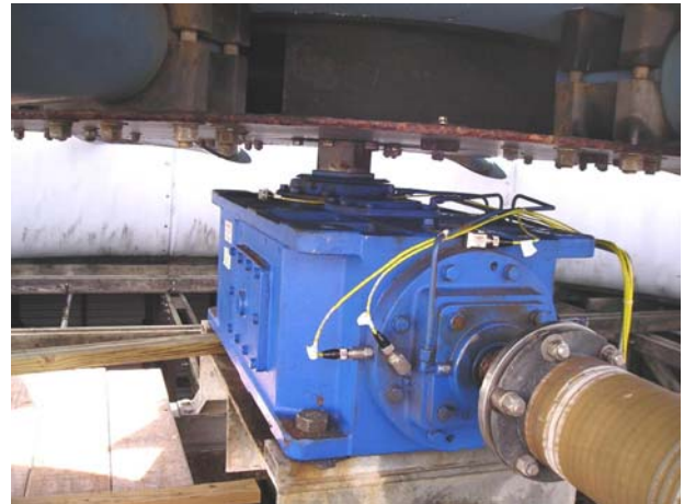
Radial & Axial Sensors on Gear Box Input Bearing Housing
